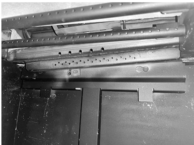
Figure 23: Remove rear baffle.
