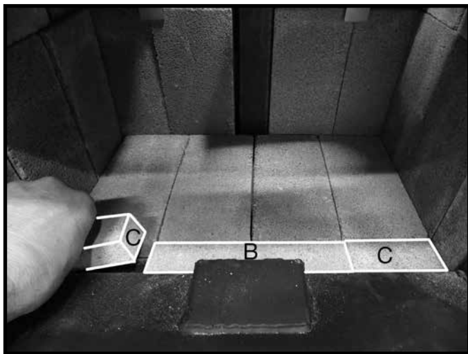
Figure 17: Narrow front bricks in place.
