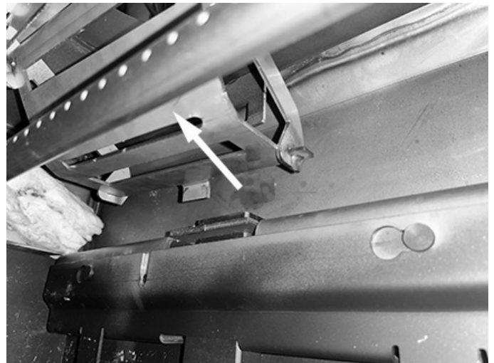
Figure 4. Remove Flue Gas Agitator.
